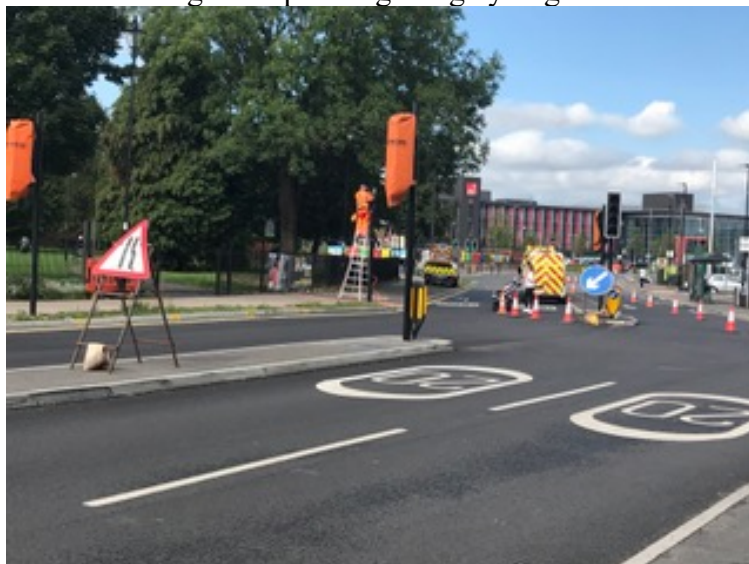
Installation of pedestrian crossing on High Street Langley near the Memorial Park Entrance
